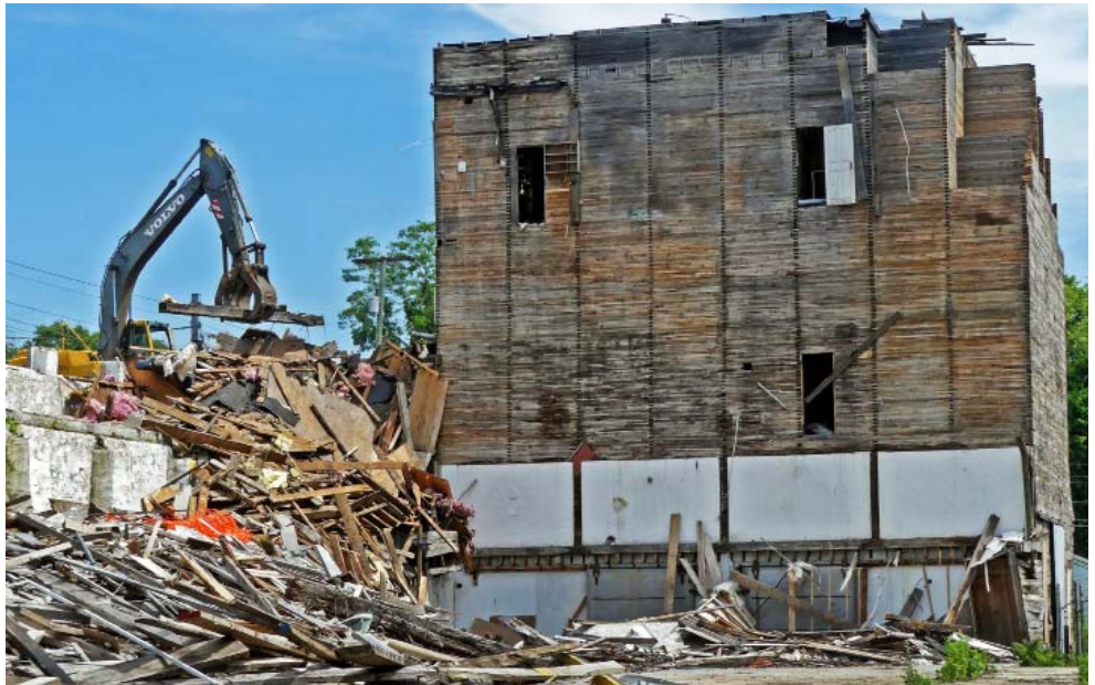
Demolition – Harold Hanka, The Westerly Sun
